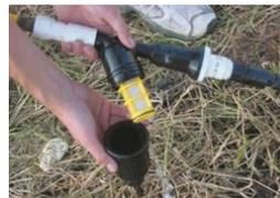
Turn on your water and let it run out the ends of the Drip tape. You never know when a little debris can get into the tape during installation.
