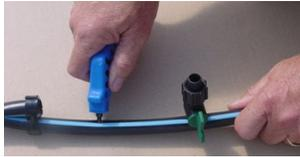
Take the Purple Punch Tool to pierce a hole where the Drip Tape meets the Poly Header. **Hold the tool against the Poly Tubing and with a pushing twisting motion, it will cut through the Poly.** Once a hole is made, take the tape fitting and push the barb into poly. Push tape onto other side of fitting and tighten nut (the same as the Power Loc Fitting).
